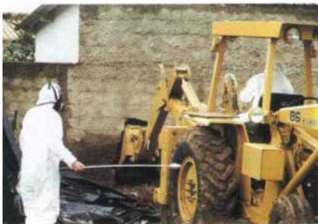
10. A hole is made to remove a radiation hot spot giving a dose rate of 0.5 \text{ Sv}\cdot\text{h}^{-2} .
