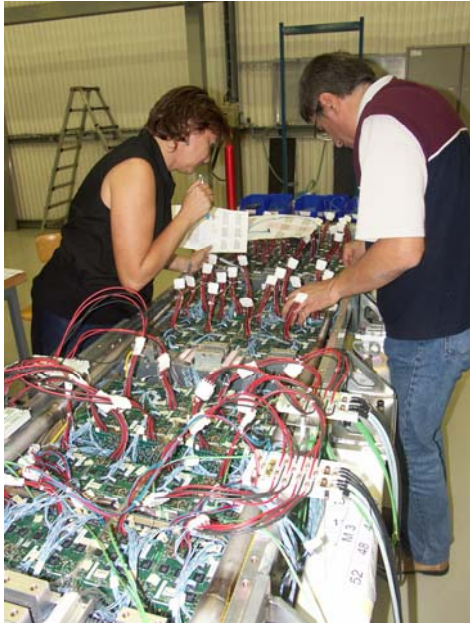
Figure 3: A supermodule after Trigger Towers and Token Rings installation.
