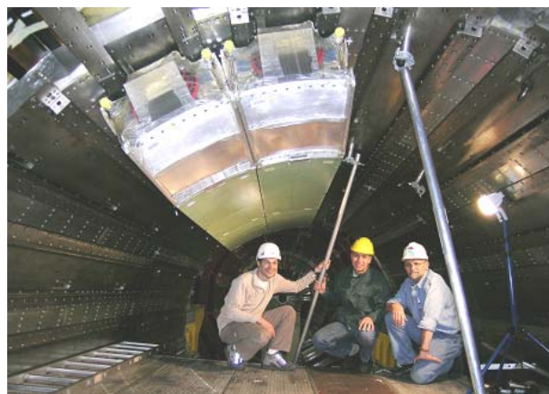
Figure 11: Two supermodules installed in CMS and the proud installation team.
