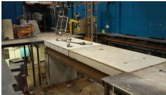
September 16: New bridge over CLEO pit
