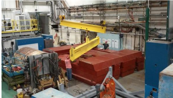
August 4: CLEO steel stockpile
