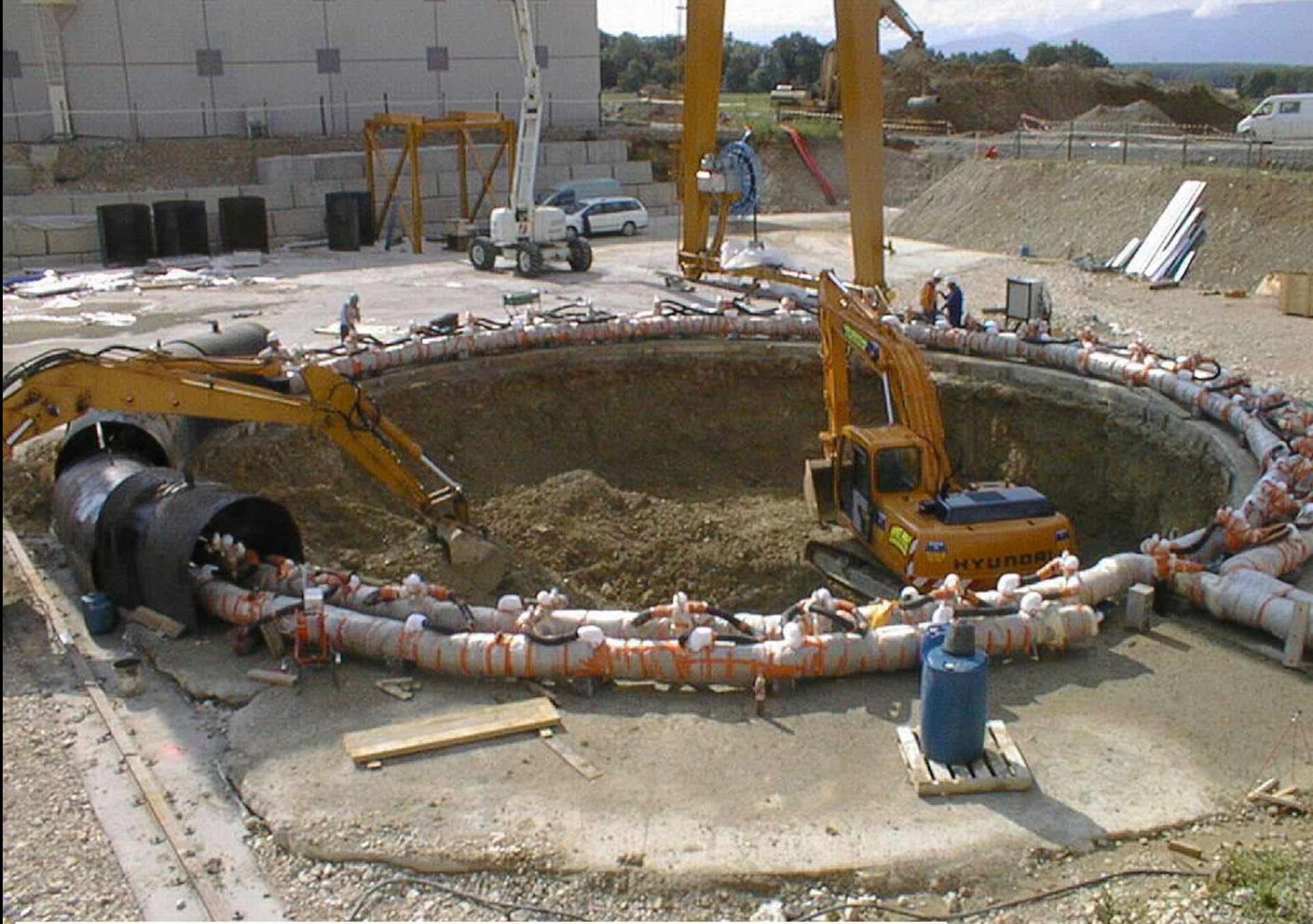
Point 5 -Excavation commencement of PM54 shaft - July 09, 1999 - CERN ST-CE
