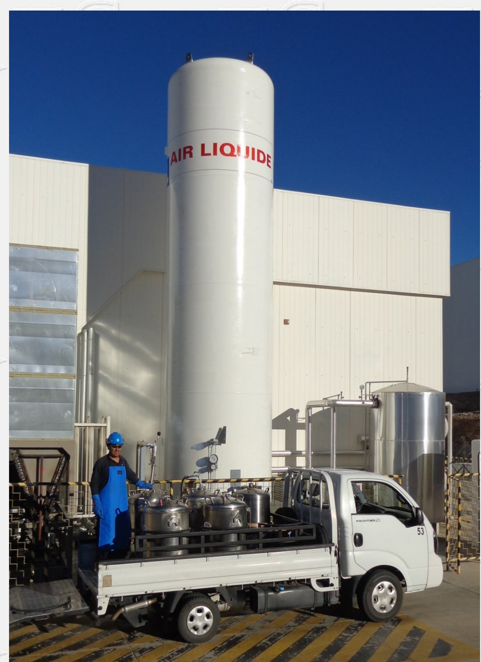
1201 tanks to deliver the LN2 toward the 60 cryogenic systems distributed over the telescope platform
