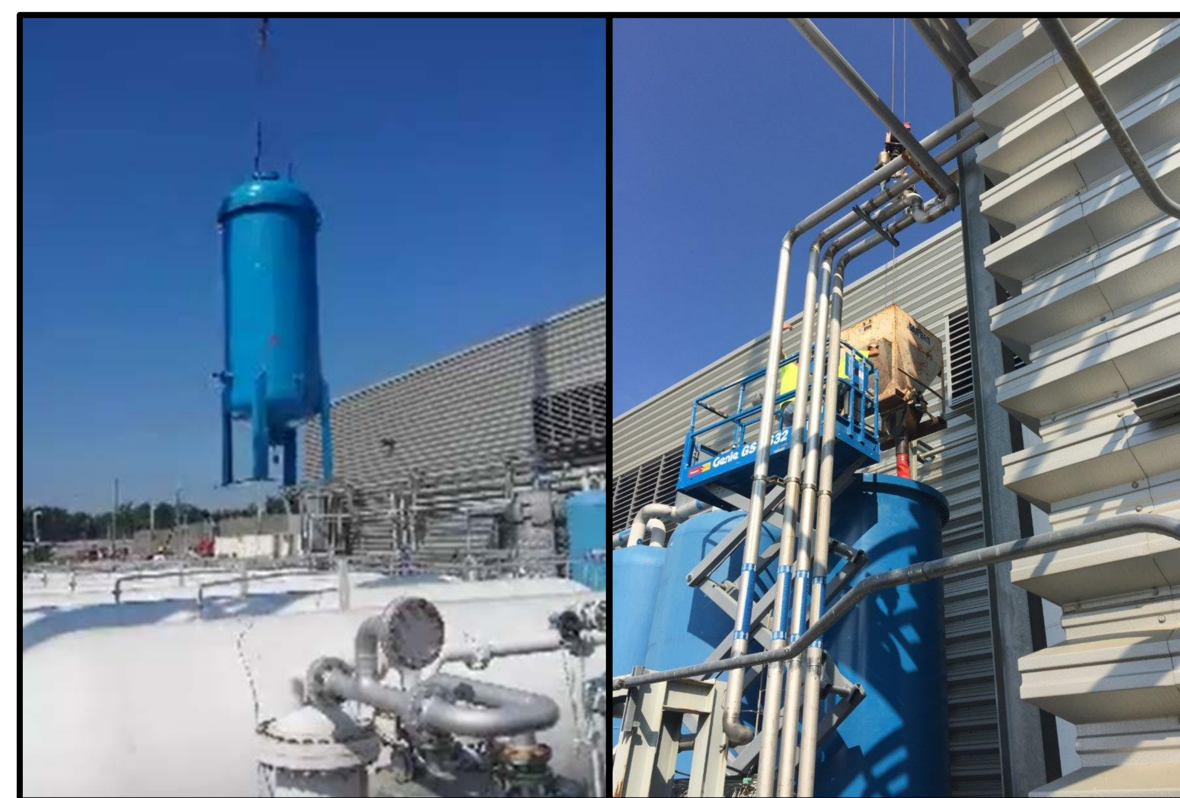
Crane Installation of Carbon Bed
