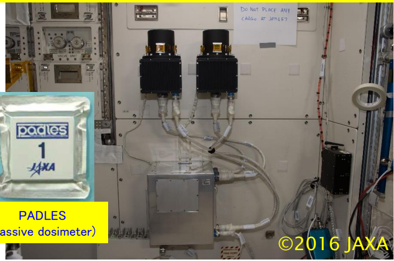
PS-TEPC installed in the Japanese Experiment Module (JEM)
