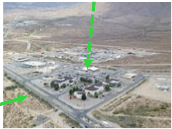
White Sands Ground Terminal, NM
