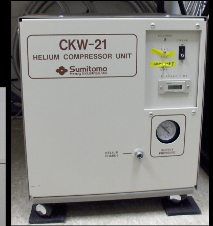
Helium compressor and cryogenerator
