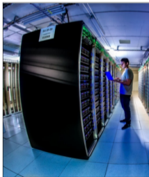
CERN's Data Centre (Image: Robert Hradil, Mo
