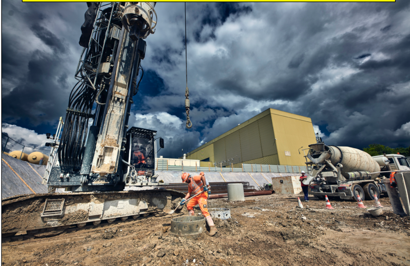
The civil engineering work for the High-Luminosity LHC gets under way. Here we see the earthmovers at work on the new 80 metre access shaft at Point 5. (Image: Julien Ordan/CERN)
