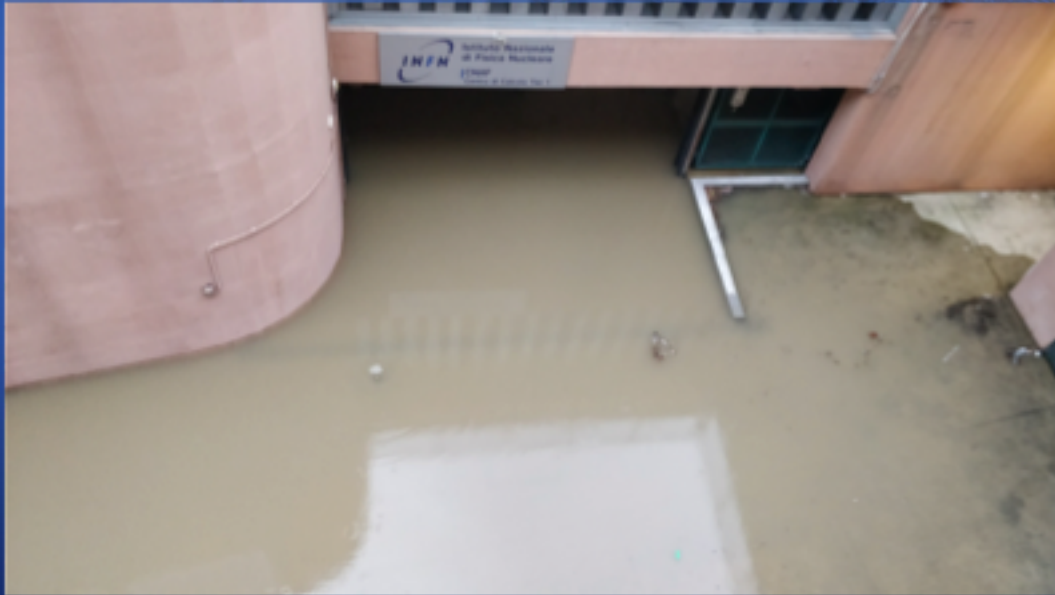
The entrance of the data center at 7.37 CET
