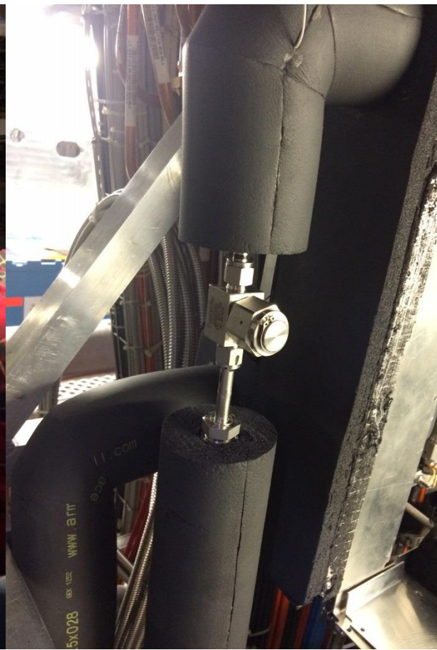
New 40um filter before IBL Manifold box
