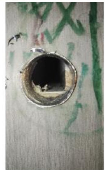
Empty gap of 10x2x95 cm in the insulation, refilled with foam
