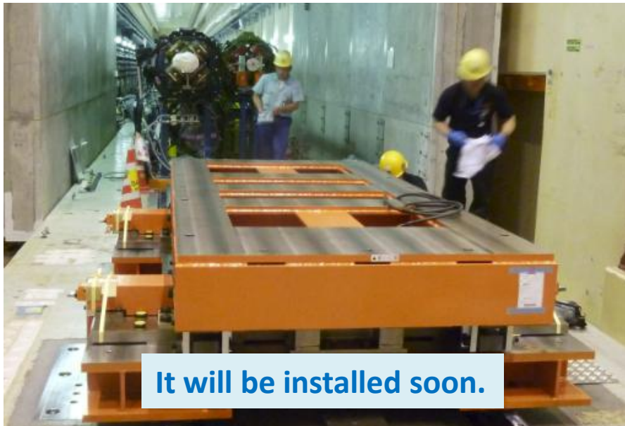
Right side of QCS (electron upstream) has been assembled.
