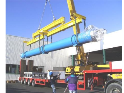
Unloading a 27 tons dipole
