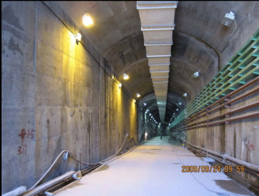
Access tunnel to the underground halls well advanced
