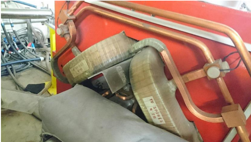
DR.QDS01 repair in-situ
