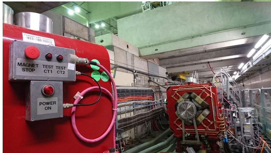
DR.BHN33 removed for renovation
