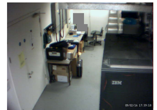
SRIF room working area
