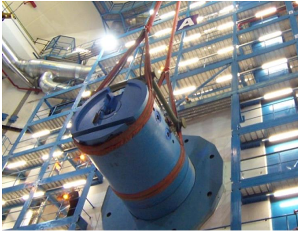
ATLAS Forward Shielding (Octagonal shielding (JFS), cylindrical shielding (JFC))
