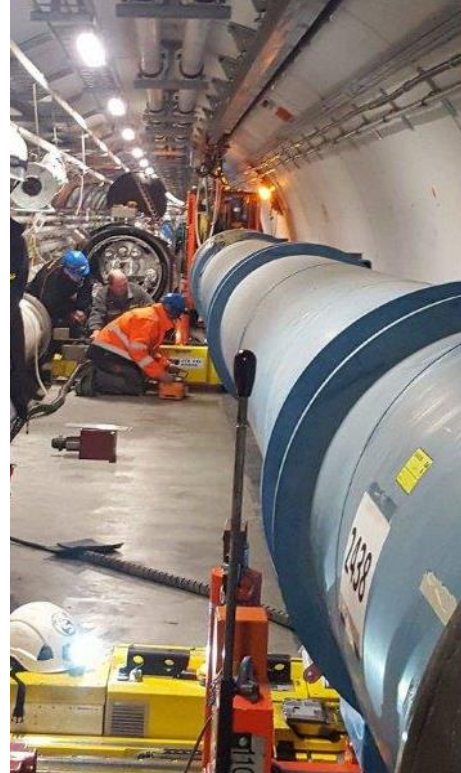
New A31L2 magnet installation
