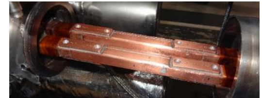
13kA splices and shunts soldered
