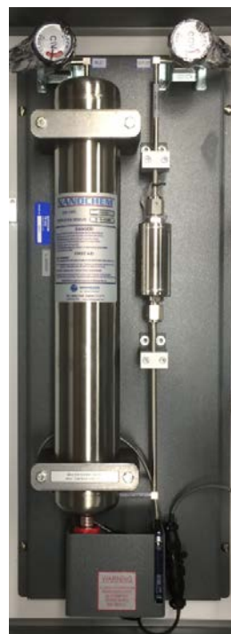
Purifier mounted into Gas Flow Control Panel
