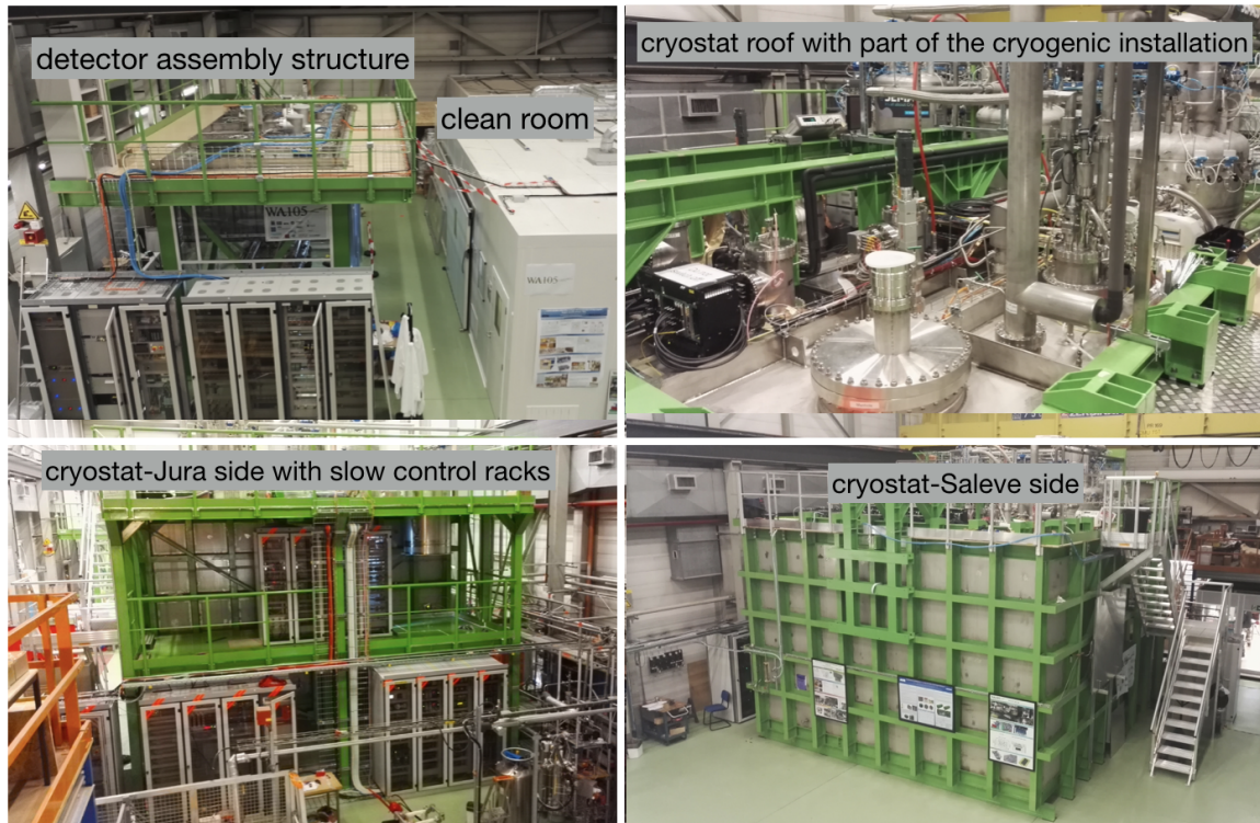
FIG. 4: Overview of the installation in building 182.
