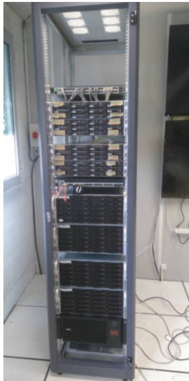
FIG. 63: Reduced scale version of the online storage and processing facility already operational for LAr-Proto.
