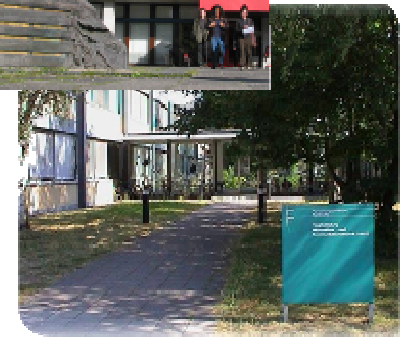
SCC at Research Centre
