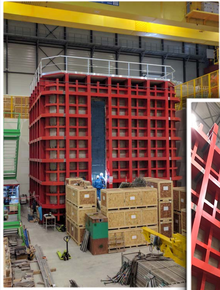
photos of ProtoDUNE-SP: cryostat external structure completed internal membrane insulation in progress
