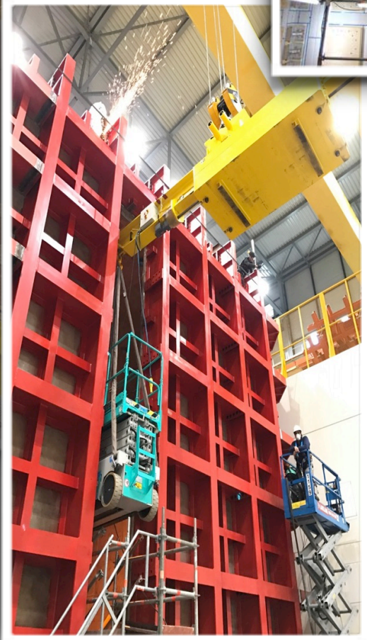
photos of ProtoDUNE-SP: cryostat external structure completed internal membrane insulation in progress
