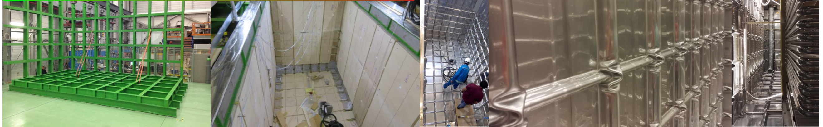
2015. 3x1x1 DP first membrane cryostat at CERN
