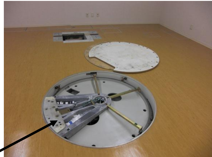
The structure of turn table in the treatment room
