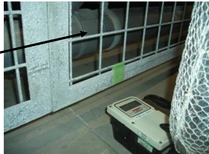
Pipes near the boundary
