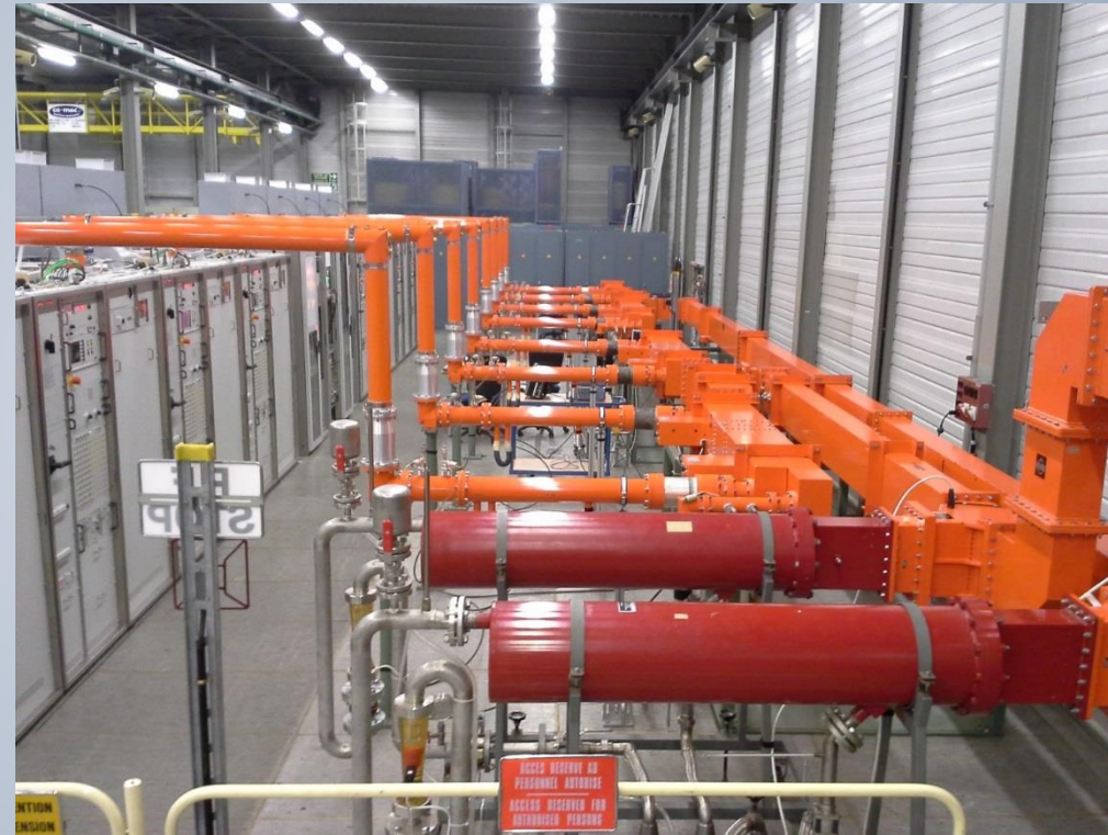
CERN SPS, TH 795 IOT, Trolley (single amplifier), and transmitter (combination of amplifiers) Two transmitters of four tubes delivering 2 x 240 kW @ 801 MHz, into operation since 2014
