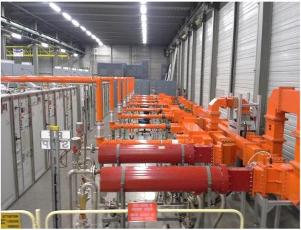
Chain of 8 IOTs installed powering two cavities in the SPS
