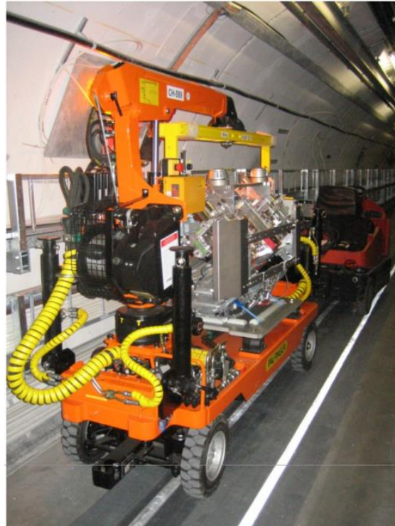
Installation – trailer/crane designed for “hands-on” use. Collimator and handling equipment designed in parallel.
