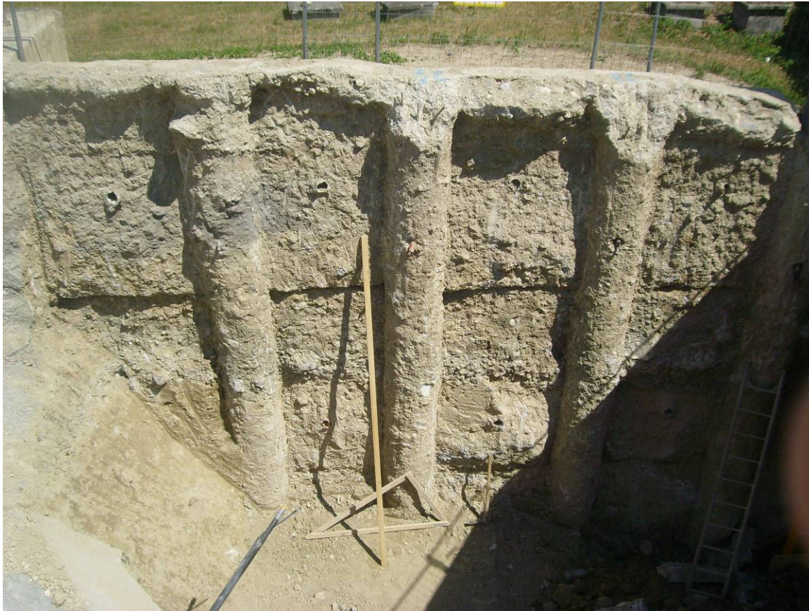
Wall of Linac2 building at connection point, 03.06.2009
