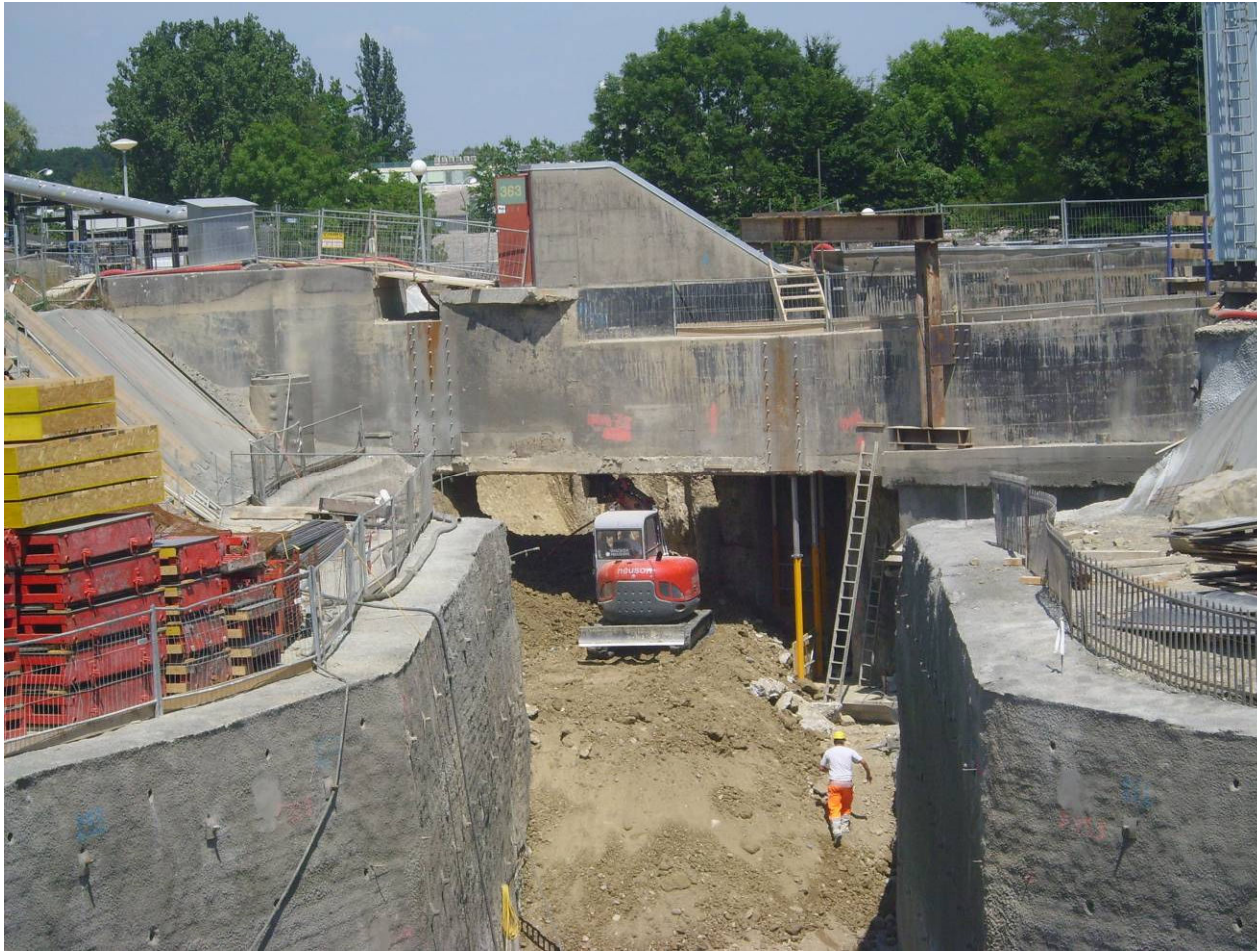
Excavation under the technical gallery PSB-Linac2, completed 25-29.5.2009
