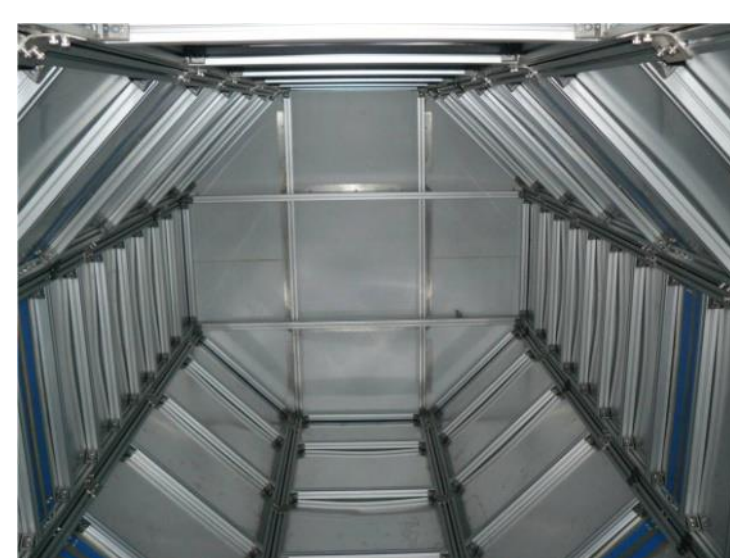
Above View from inside the scaffold, after panels have been fitted on.
