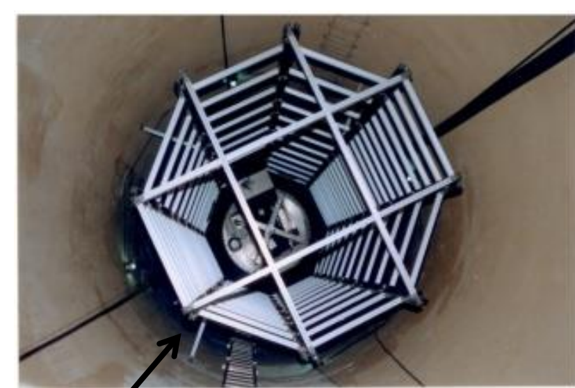
The scaffold, built with extruded Alum. Profiles for ease of fitting and modularity. As installed in Underground Laboratory
