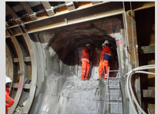
Crossrail – Cross Passage Temporary Frames
