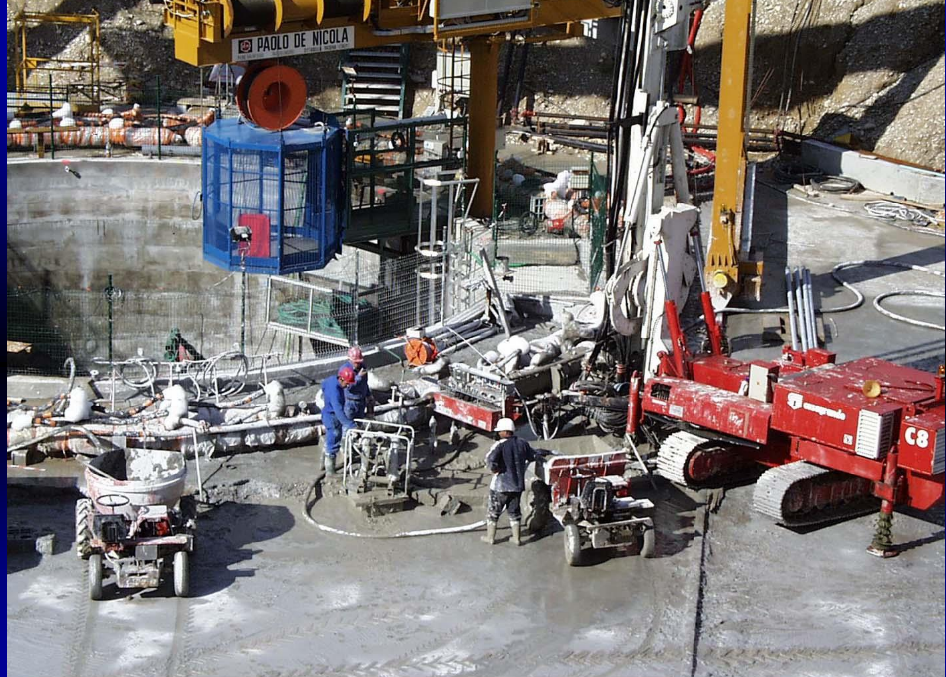
Point 5 - PM54 additional drilling for grouting - October 01, 1999 - CERN ST-CE
