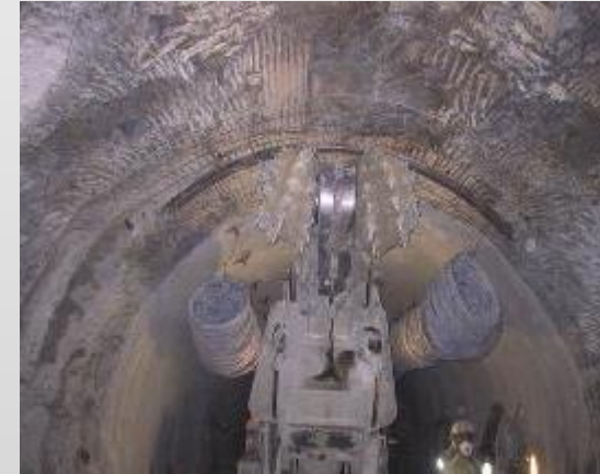
Roadheaders will be used for excavation
