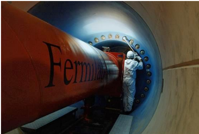
Access to Q1 extremity into the shielding
