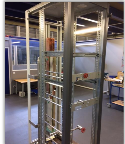
The busbars and the cooling water pipes are installed
