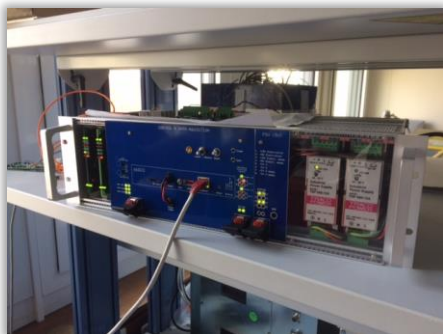
3U control chassis housed the electronic boards
