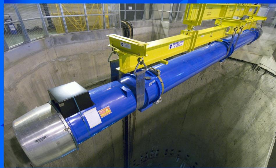
Main Dipole – transfer to the installation point
