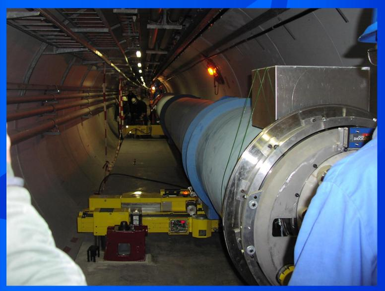
**TES** – Main Dipole placed above support jacks, checking process for correct position of support jacks versus support plate holes.
