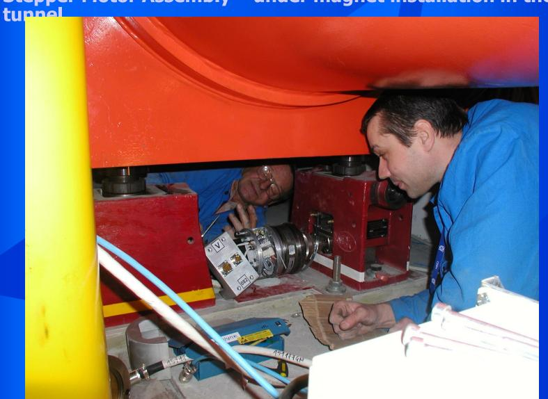
Stepper Motor Assembly — under magnet mechanicall calibration
