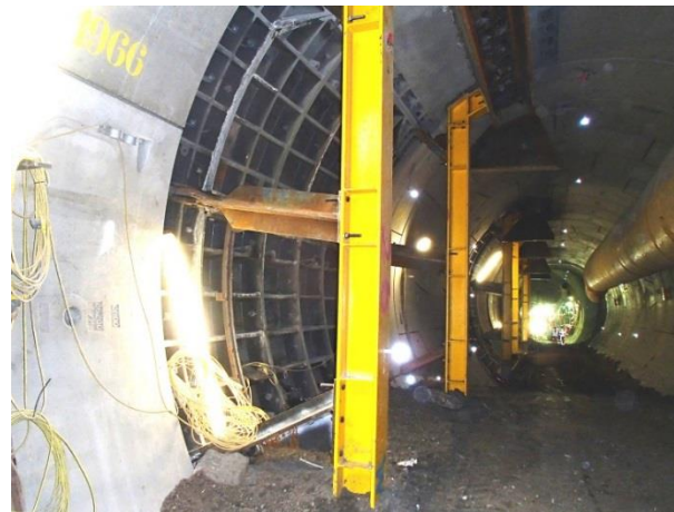
Crossrail – Cross Passage Temporary Frames
