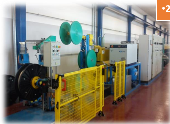
20 meter long in-line furnace
