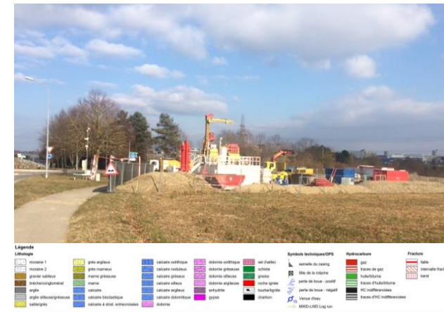
Geothermal site investigation in Satigny 2017/2018 (500m deep)
