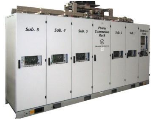
CERN's 13kA-18V LHC dipole converter.
