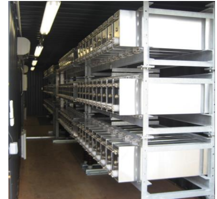
Capacitor bank used for the powering of PS.
