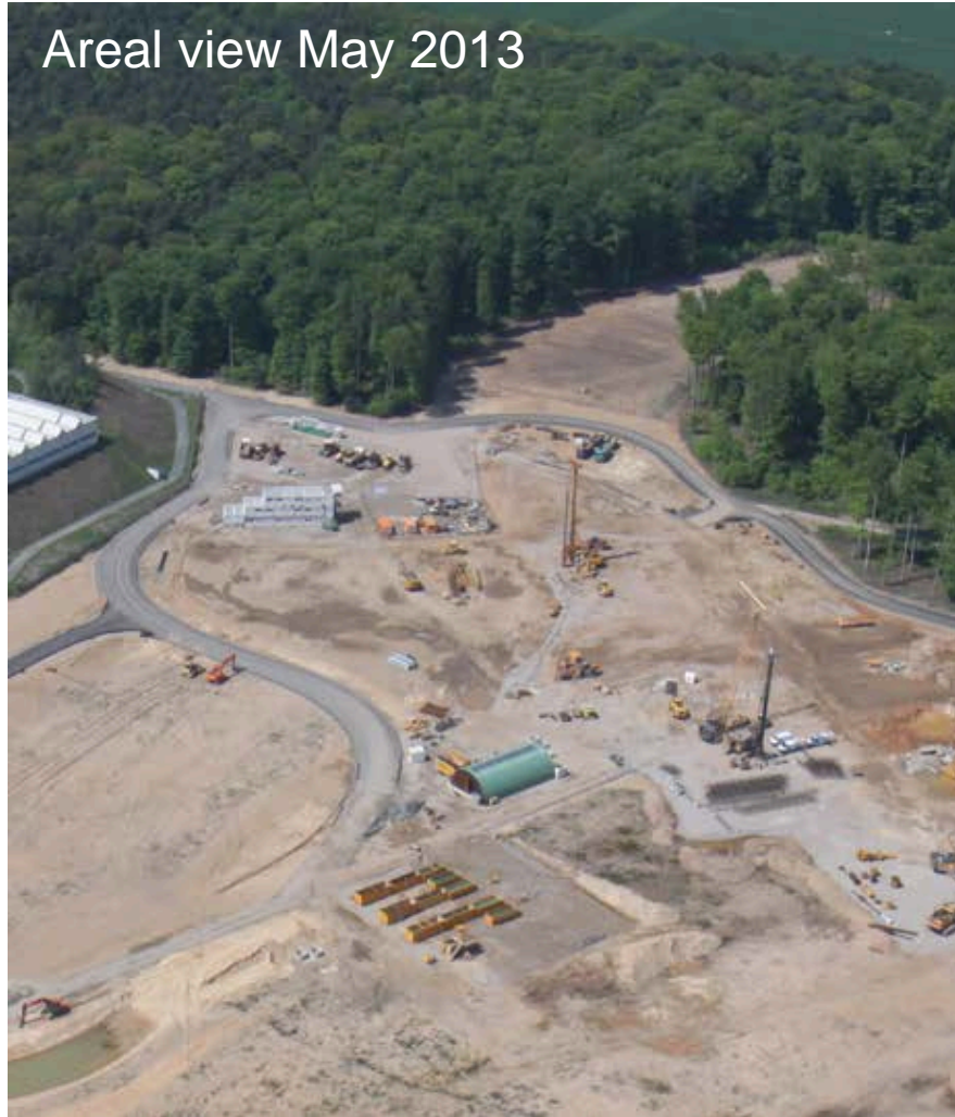
About 500 pillars erected
