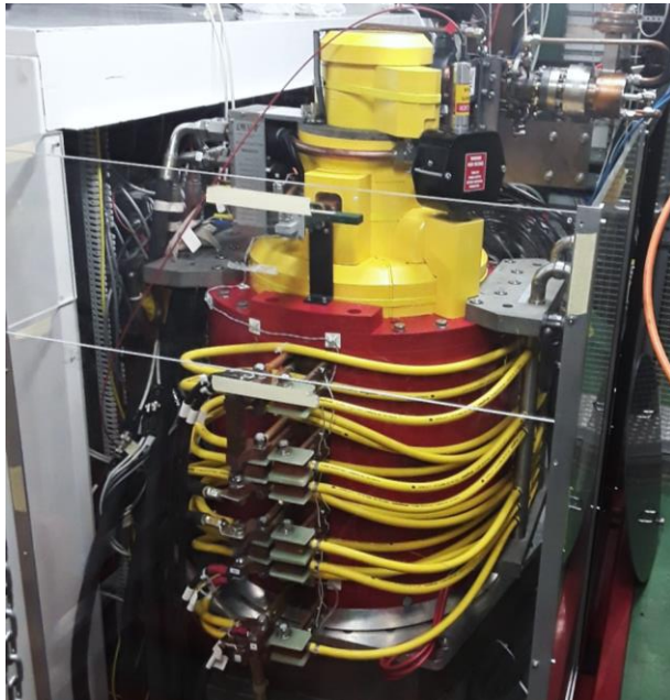
New XL5 klystron installed in modulator. Waiting the CPI team.
