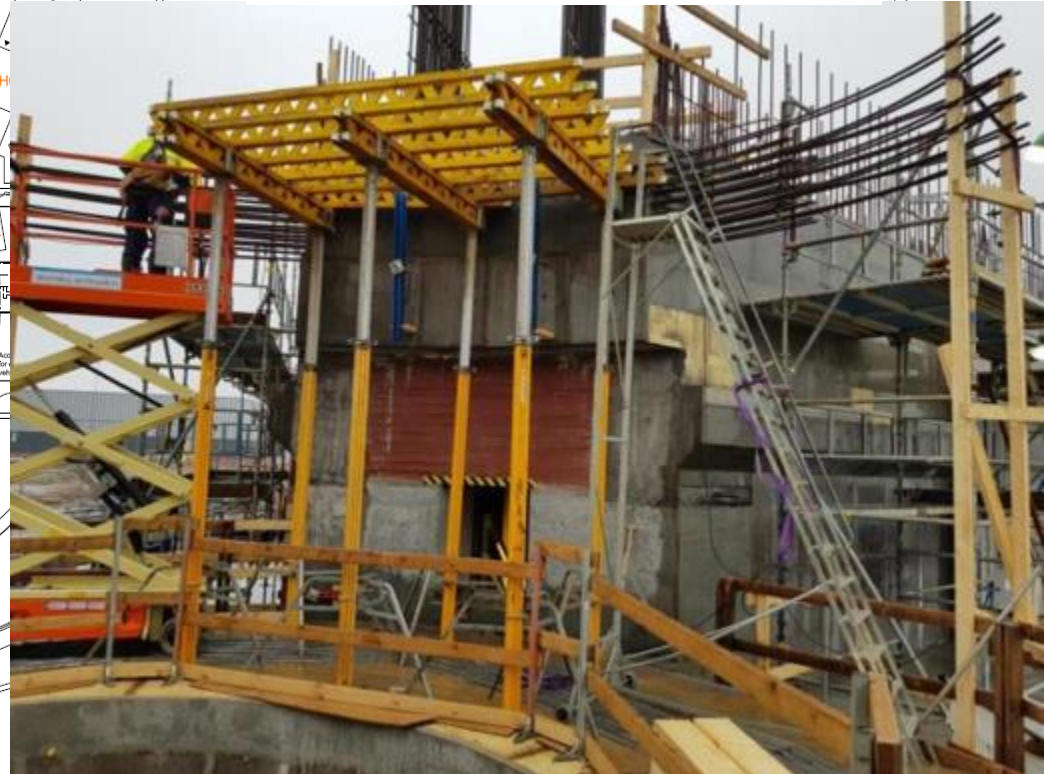
Shielding plates installed
