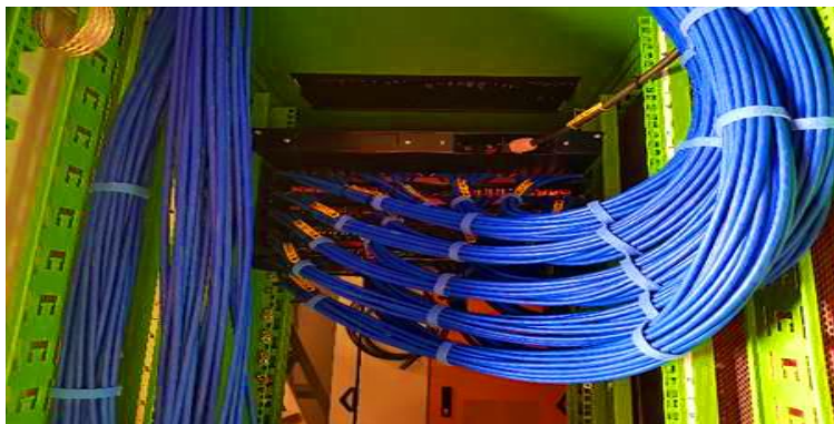
Cabling on site
