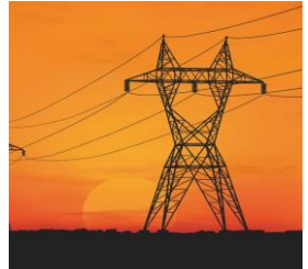
Fault current limiters
