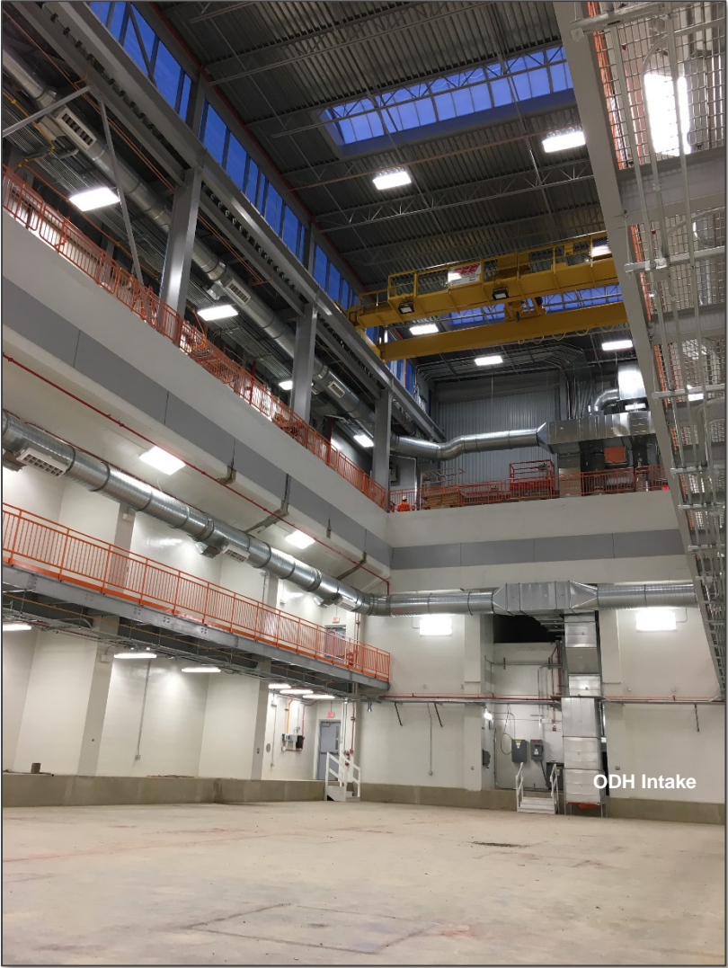
Looking North From Enclosure Level
