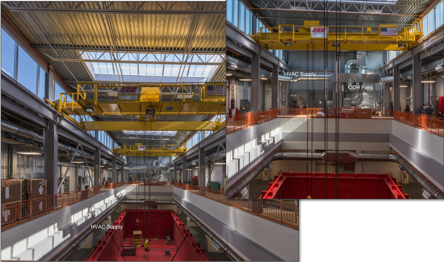
Looking North From Loading Dock
