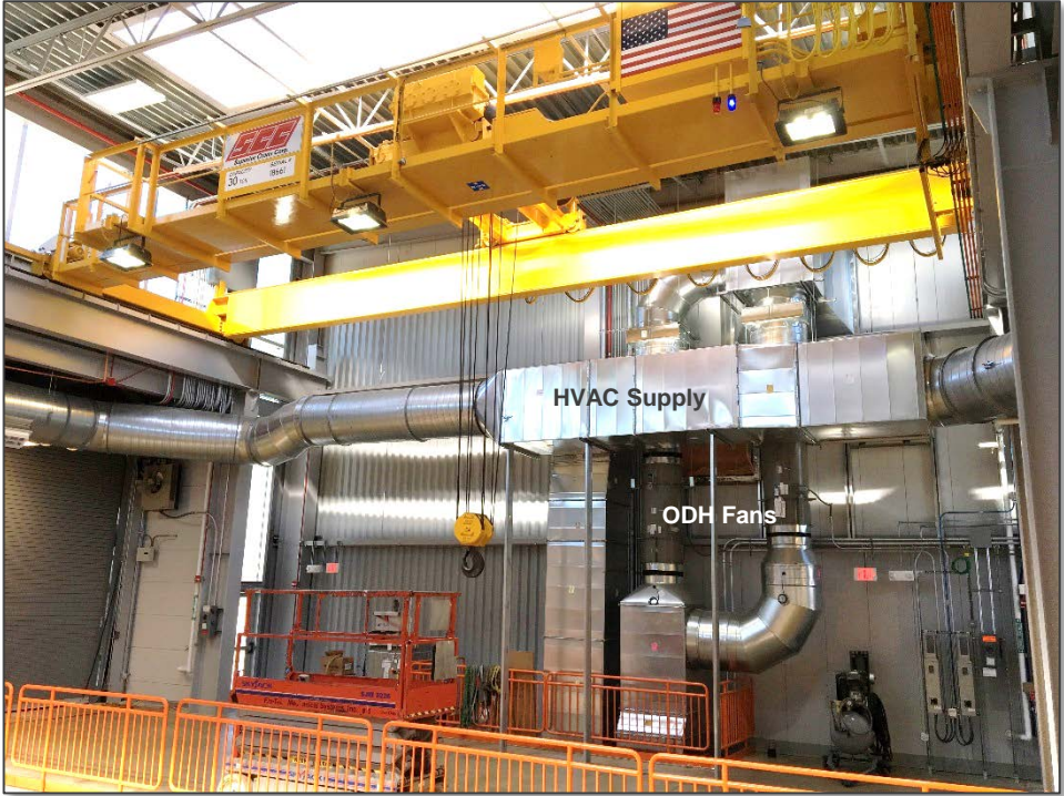
Looking North at North Wall
