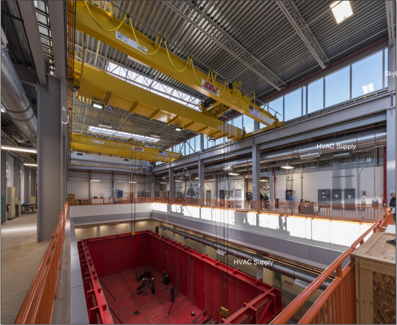
Looking South From Loading Dock
