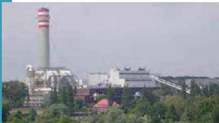
Fig. 4.15: A pilot flue-gas treatment plant in Poland using an electron-beam accelerator to remove pollutants.
