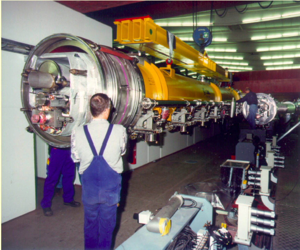
Cryomodule installation in the tunnel (the XFEL consists out of 101 cryomodules)
