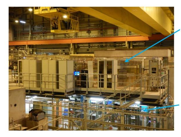
First floor: gas service area. ~ 20 gas racks and distribution panels (40 m<sup>2</sup> net area)
