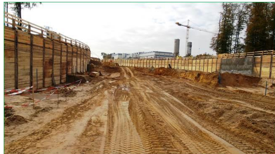
Excavation SIS100 tunnel - Nov 2017
