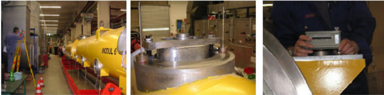
Figure 70: Measurement of vessel and setting of side panel
