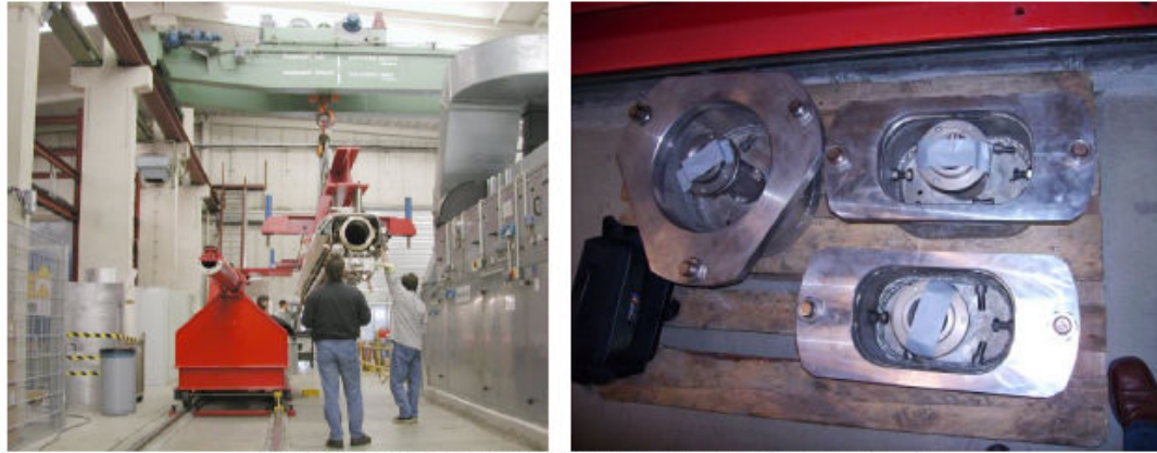
Figure 50: Transport to cantilever and disassembled posts
